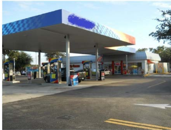
Example of Typical Canopy Serving Fuel Stations
